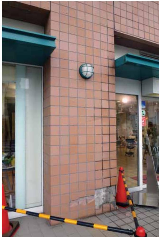
**Figure 5.** Minor spalling at the base of the columns of Namagachi Lions Tower.
