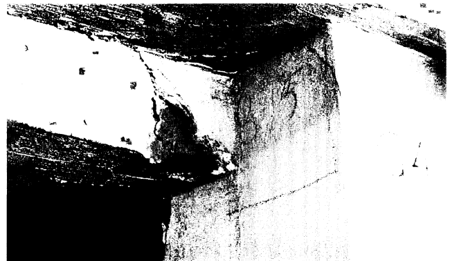
Fig. 4 — Cracks at column G4.
