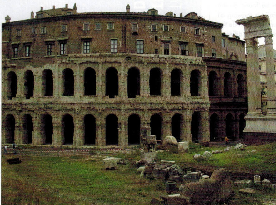
Fig. 1: Prefabrication and in-situ construction have always coexisted. In the case of the figure, they belong to different times but to the same building: Roman Teatro di Marcello with Renaissance Orsini Palace on top of it.
