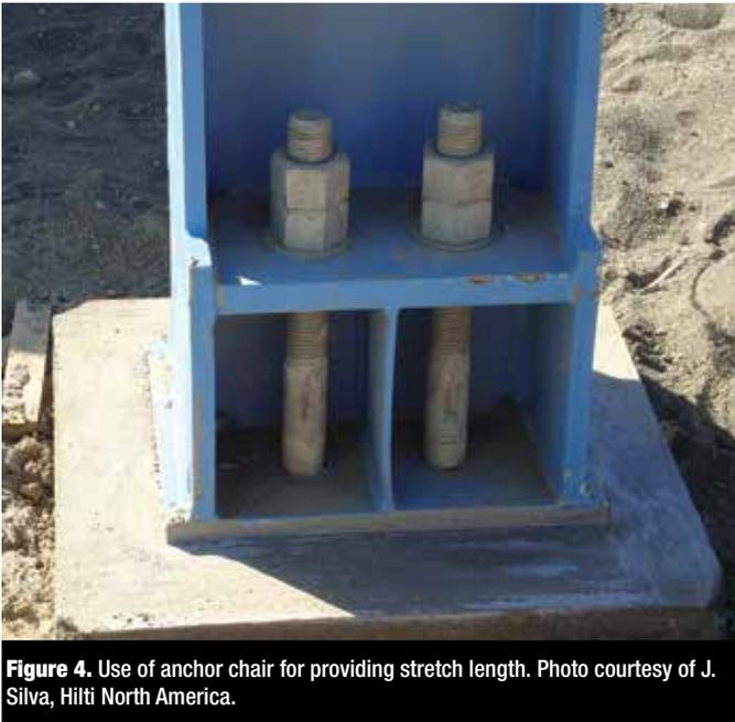
**Figure 4.** Use of anchor chair for providing stretch length. Photo courtesy of J. Silva, Hilti North America.
