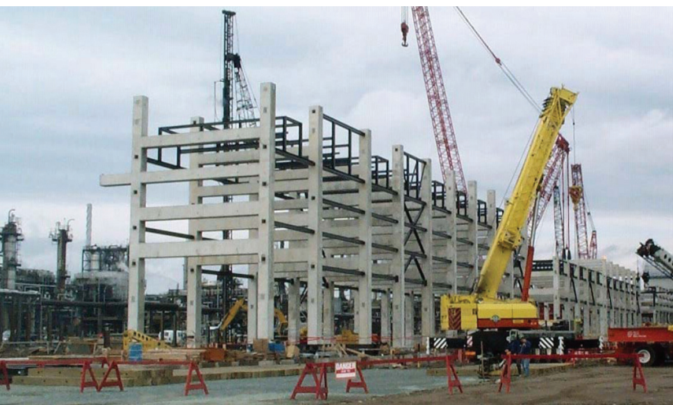
Nonbuilding structure similar to a building.
