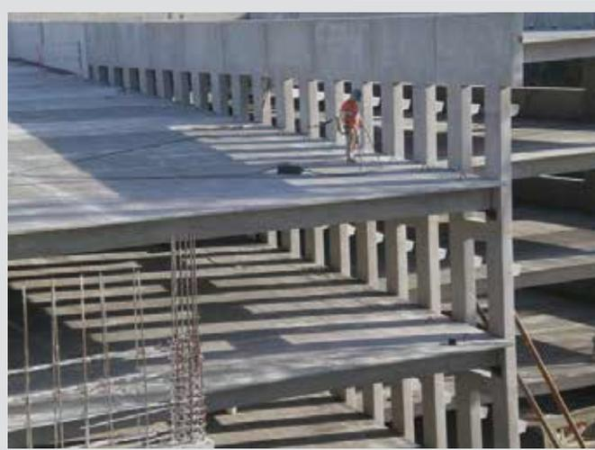
**Figure 3.** Precast concrete double-tee deck diaphragm. Image courtesy of Pat Hynes, Knife River Prestress Division, Harrisburg, Ore.
