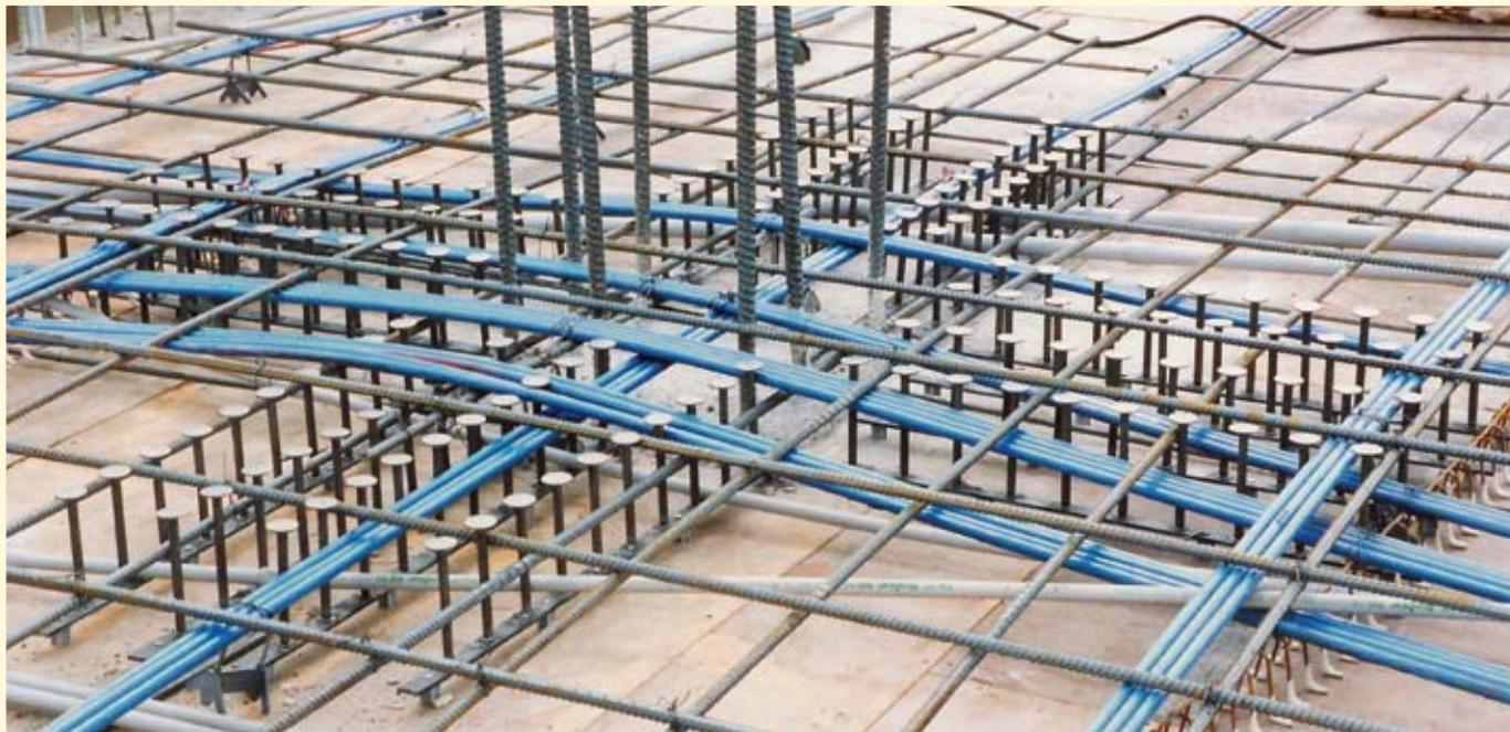
**Figure 1.** Stud rails are used as slab shear reinforcement. Photo courtesy of Decon U.S.A. Inc.
